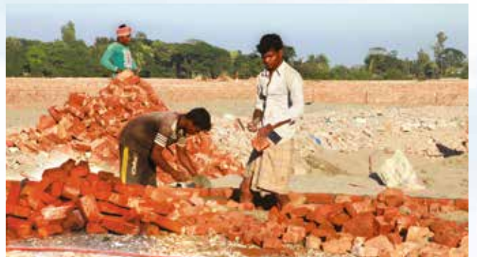
ONGOING PLOT BOUNDARY BUILDING
