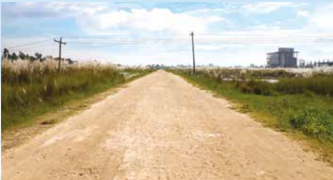
164 FEET WIDE ROAD WORK IN PROGRESS
